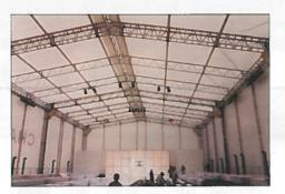
presentation, Faber Image would be in possession of an eight-mast tower system and substantial quantities of the safest truss available." There were other benefits for Faber Image: the structure is designed to be free standing and is still rated for 25 m/s winds and a four-tonne payload. Thanks to its design, it can easily be split into two separate, fully-enclosed units, and it requires no cranes or heavy lifting gear to put it up.
