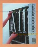
Each individual six circuit module can be set for dimming or switching operation.
